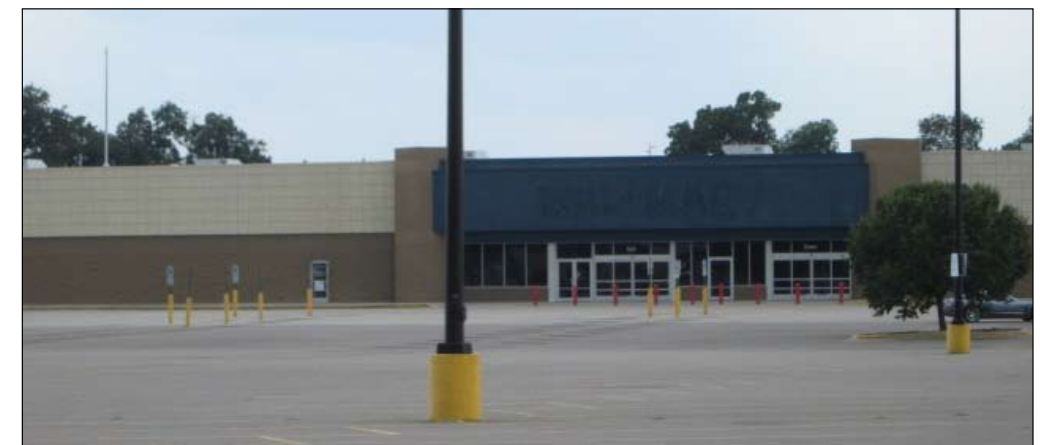
Existing Vacant Big Box Along Ramsey Street
